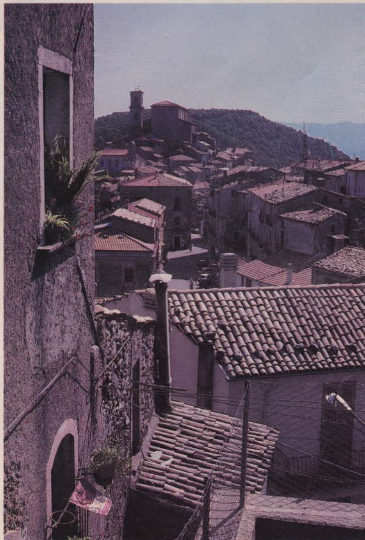
San Fili, a gentle mosaic of red-tile rooftops and gray walls against a backdrop of mountains, had changed little since the author first saw it 14 years ago.
